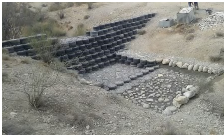
Figure 1. Rubber Dam in the evaluated cases.
