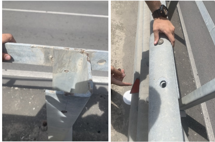
Figure 13. Use of welding in road guardrails.
