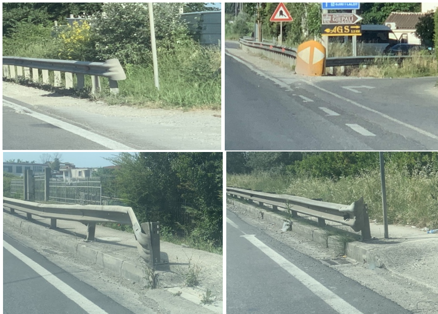
Figure 14. Ending elements of road guardrails.
